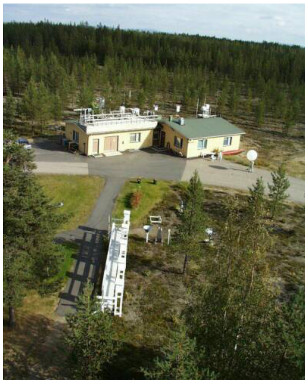
Figure 1. View of Sodankylä observatory. The Brewer is located on the roof in the enclosure on the left.
