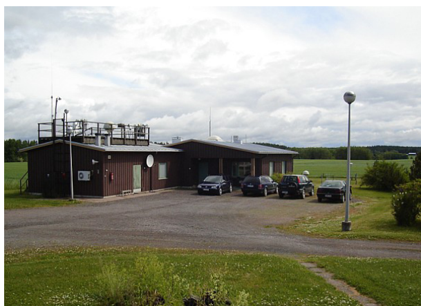
Figure 2. View of Jokioinen observatory. The Brewer is located on the roof in the enclosure on the left.
