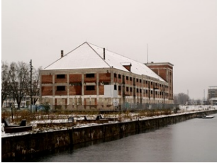
Fig_2_ The empty Entrepôt Seegmuller in 2010. Source: photo by Pierre Rudloff from Wikipedia, public domain
