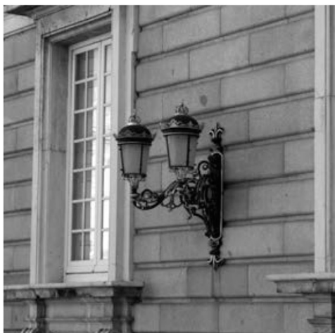
Figure 1. Farol at the Plaza de la Armeria in Madrid, Spain (from Guerrero Fernandez, 2009 ).
