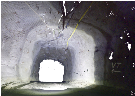
(a) Inside view of a tunnel
