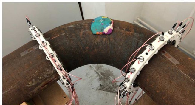
Fig. 3. The mean and the standard deviation of the fouling map reconstruction distribution on the unraveled pipe bend (upper row). 3D visualization of the fouling map (middle). The round plasticine patch of 10 cm diameter was placed on top of the pipe bend (lower).
