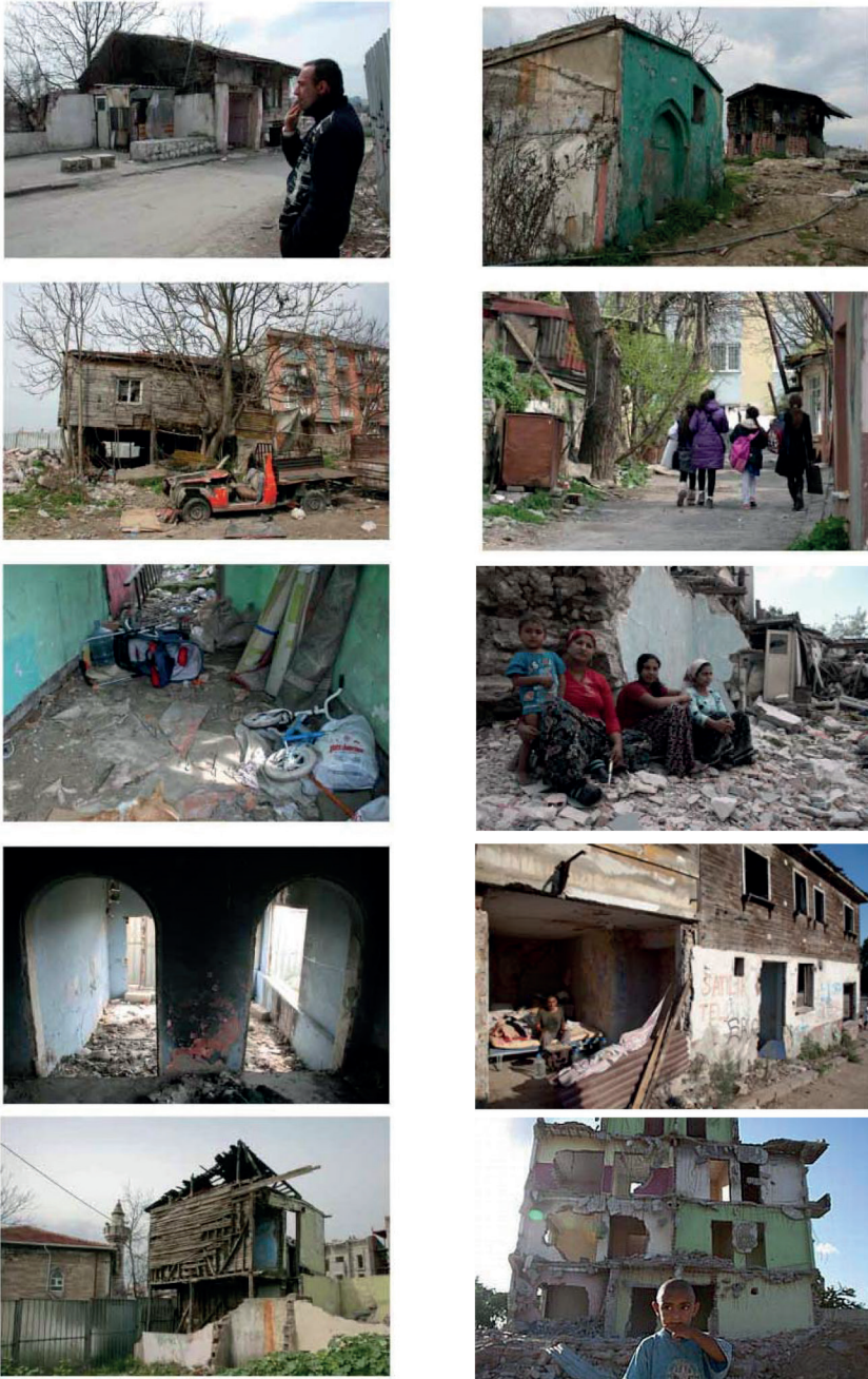
Figure 3 Some of Sulukule's Romani dwellers continued to live in the neighbourhood during and after demolitions (Courtesy of Abdullah Agah Öncül and Jonathan Lewis).
