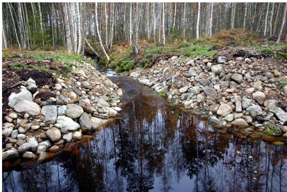
Figure 9.3. Submerged weir of forestry (Samuli Joensuu).
