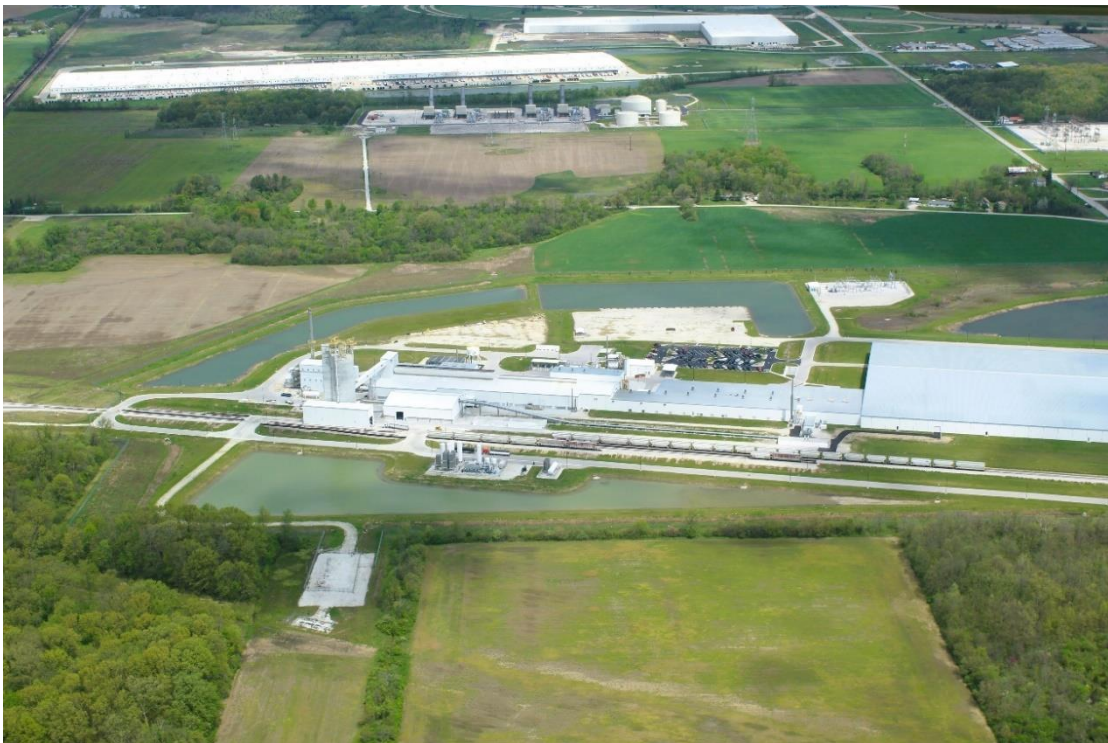
Figure 8: NSG Glass (bottom structure) and the Troy Energy Facility (top structure), a 796MW Gas Fuel Oil power plant providing heat and energy to the factory, 2024. Photo: Authors
