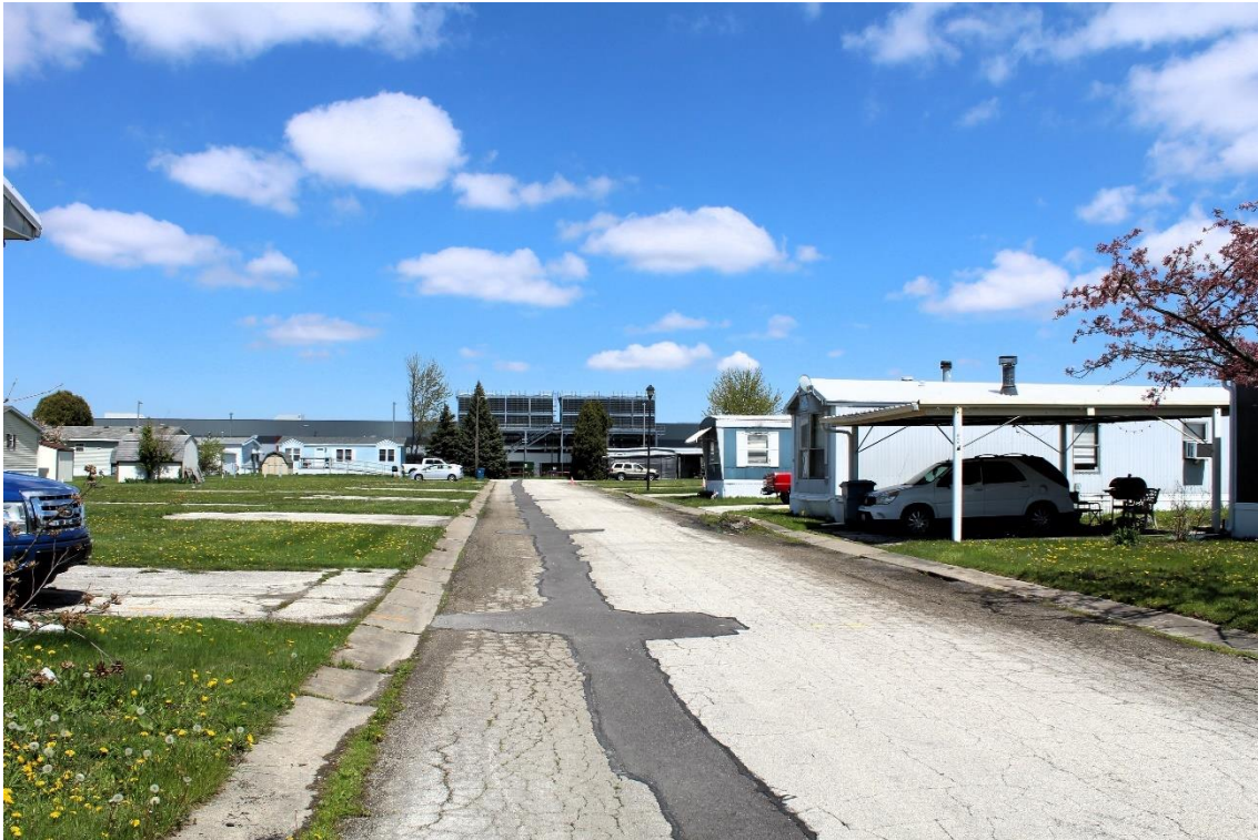
Figure 5: R&D Facility under construction seen from another vantage point in the Friendly Village Estate, 2024. Source: authors
