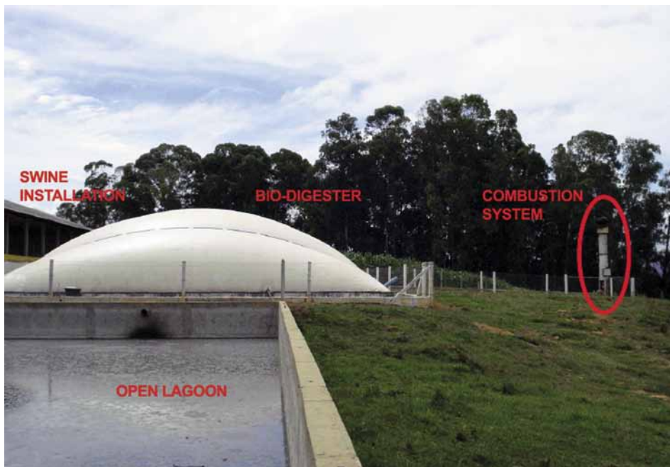
Figure 2.3 View of the biogas system (from CDM-SSC-CPA-DD Version 1, 3S Programme)
