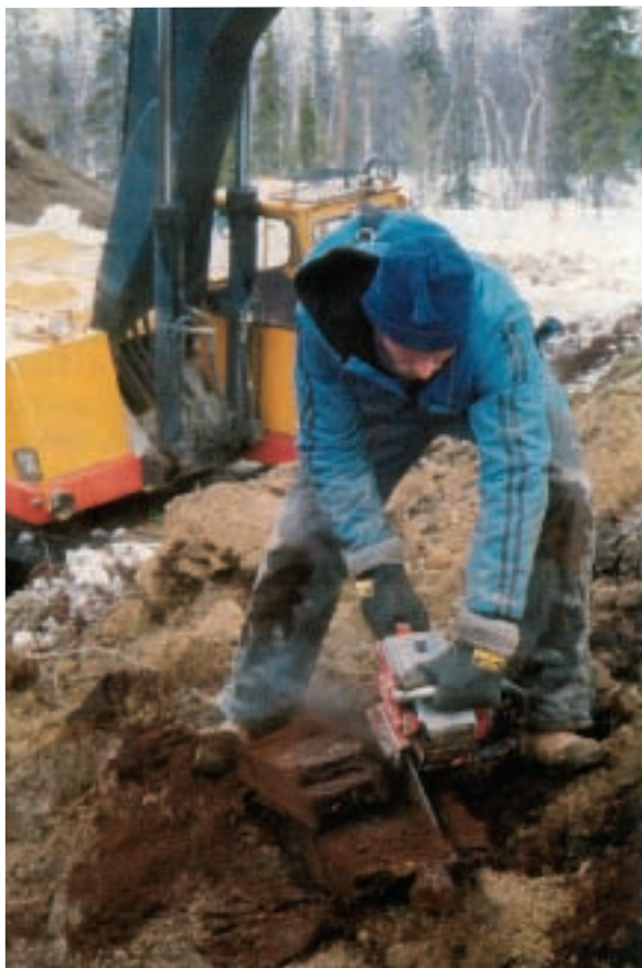
Fig. 10. The sub-till peat at Naakenavaara was so tightly compressed and hard that it had to be cut with a chain saw. Photo: Heikki Hirvas.
