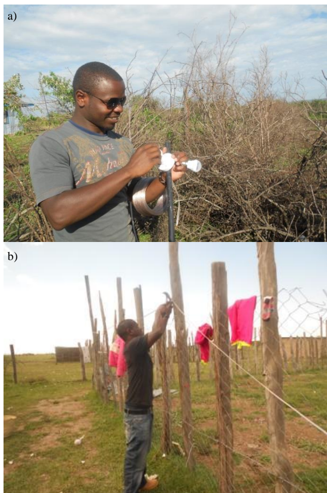
Figure 1. Installing LED lights at a boma: (a) fixing bulbs to a pole, (b) fixing a boma with connecting wires
